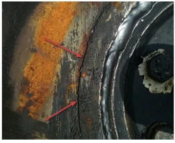
Failure of the internal cross members can lead to externally-visible cracks around the welds between the king pin retention plate and the skid plate.
